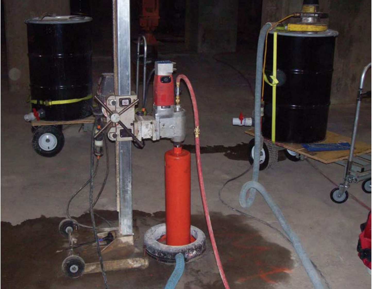
Core drilling floor holes for anchors.
