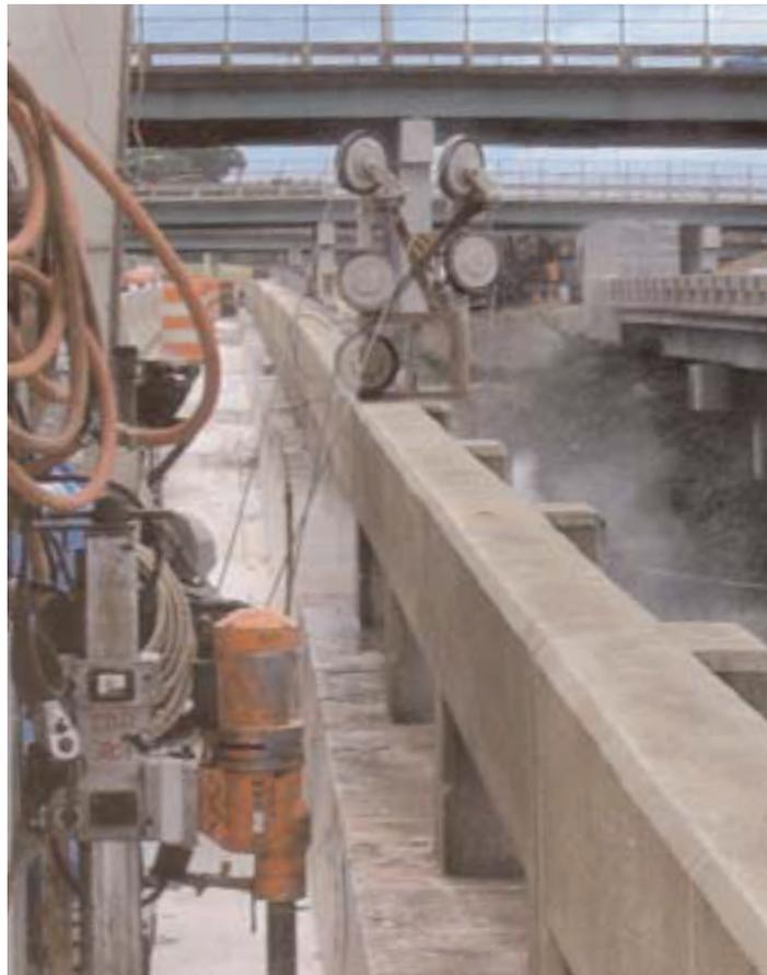
Bridge rails were cut into 50-foot sections to be removed by crane.
