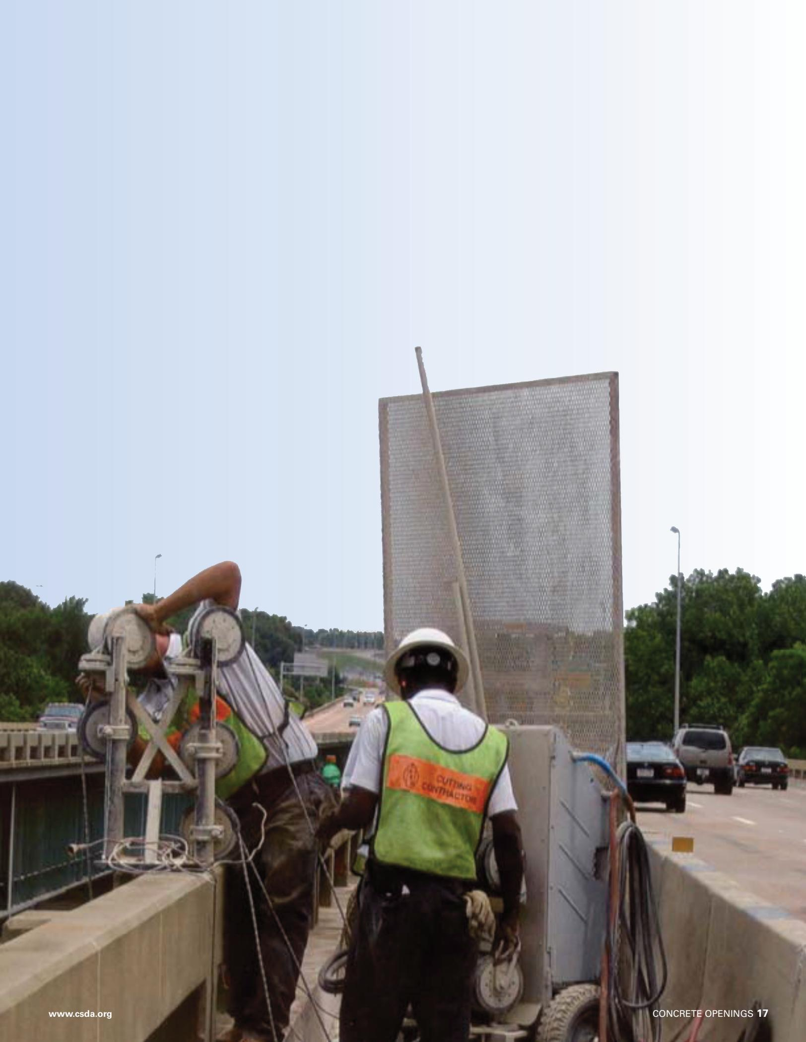
debris. In May 2006, CSDA member ABC Cutting Contractors of Alabama won the bid for the removal of the existing 9-inch thick concrete bridge rails using diamond-cutting technology.
