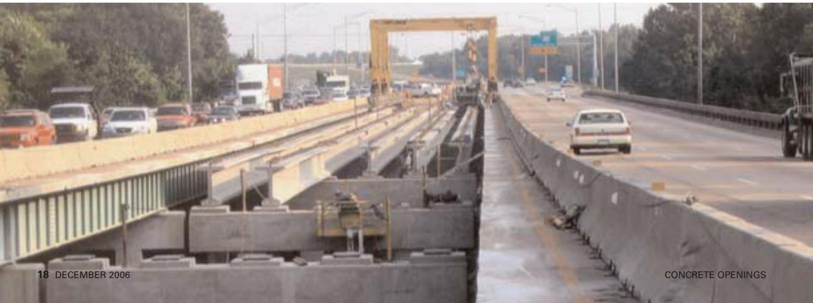
the flat saw to finish cutting the 10-foot sections. As each section was cut, each 50-foot long bridge rail section was released from the bridge. The crane holding it would then lower it to the ground.
