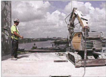
True-Line Coring and Cutting safely brings down three silos and a grain elevator at the Port of Tampa using remote-controlled Brokk machines.
