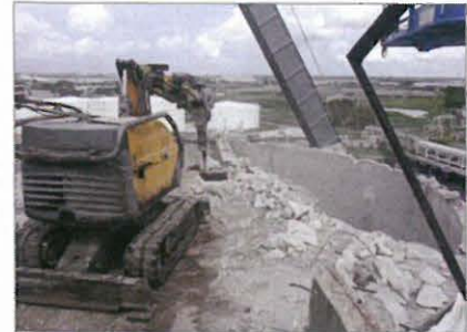
True-Line Coring and Cutting safely brings down three silos and a grain elevator at the Port of Tampa using remote-controlled Brokk machines.
