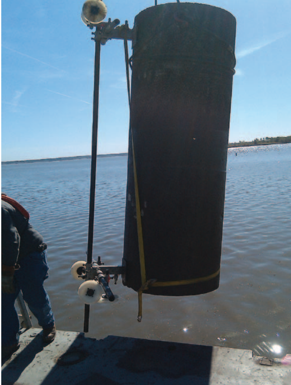
Cut sections weighed an average of 21,000 pounds.
