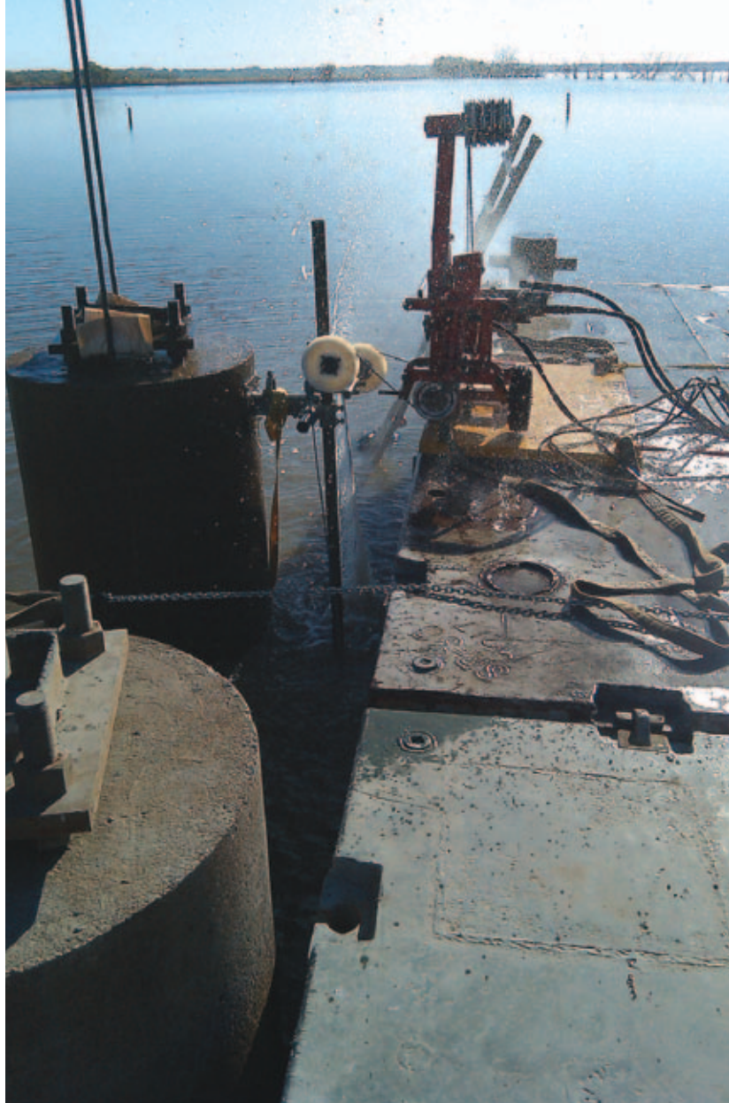
Each 4-foot-diameter pier took three hours to cut.
