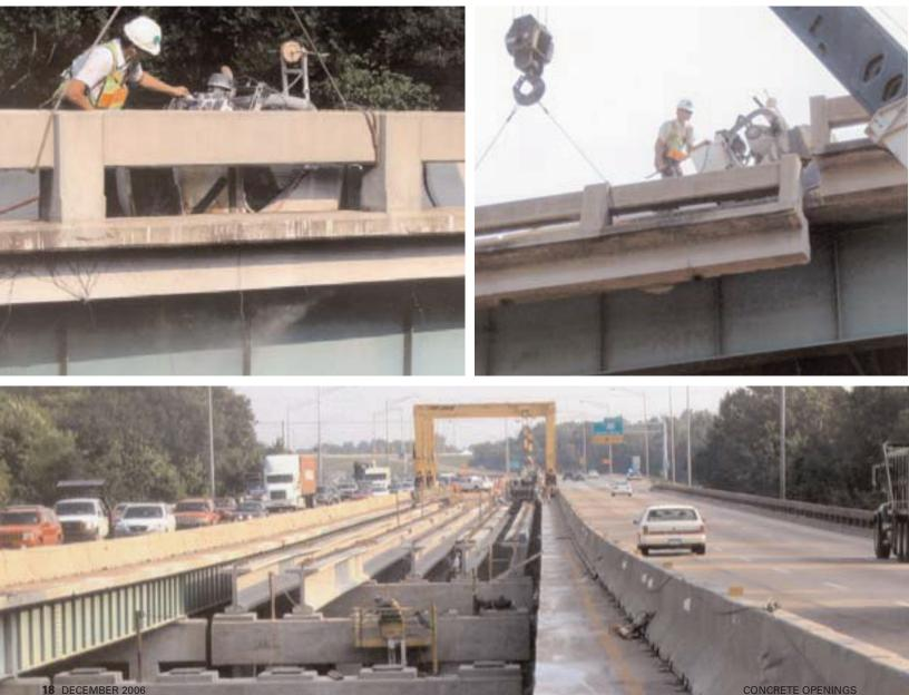
the flat saw to finish cutting the 10-foot sections. As each section was cut, each 50-foot long bridge rail section was released from the bridge. The crane holding it would then lower it to the ground.
