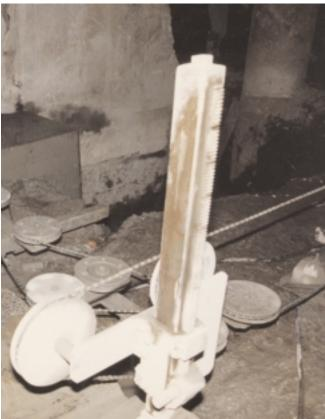
Top: The TVA Cumberland City Fossil Plant was built in the 1970s and required renovations to reduce emissions. Left: Wire sawing was a critical factor on the TVA job, especially when removing large sections of concrete. Wire sawing was much faster cutting, reducing cutting time by one-third.
